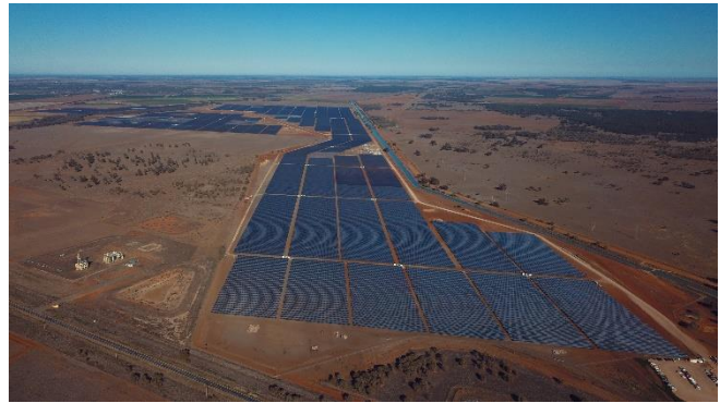
Figure 21: Coleambally solar farm. Source: Bouygues Construction
