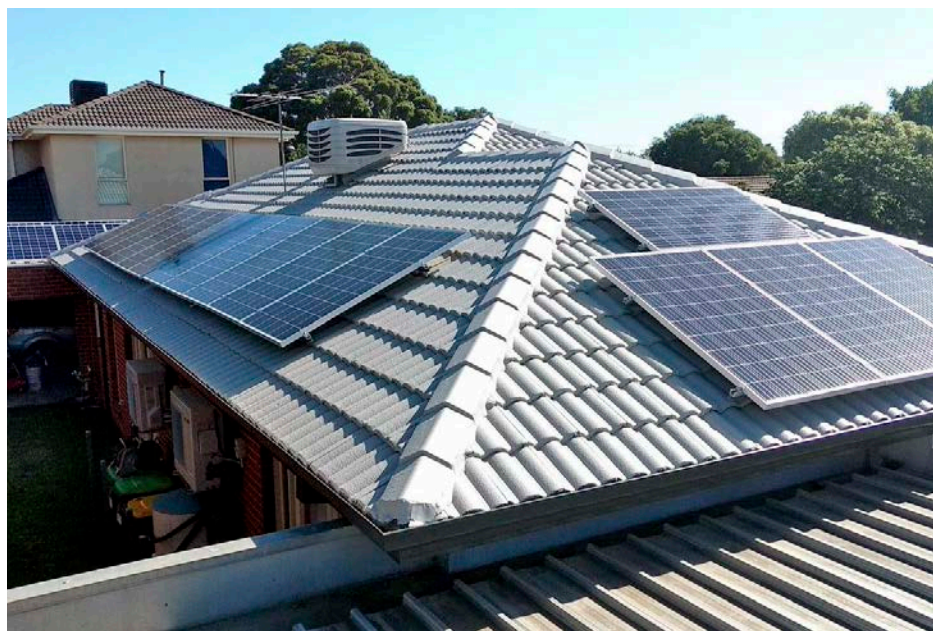
↑ East- and west-facing roofs are still fine for solar installations, if shading is at a minimum.
