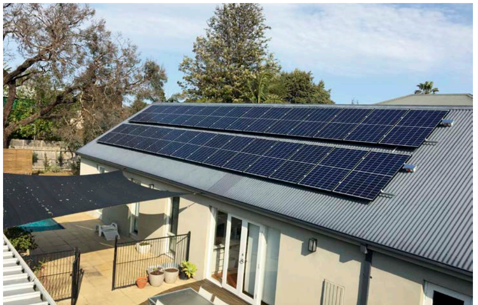
Solar systems now tend towards larger sizes, with the average size being around 7kW and many closer to 10kW.
