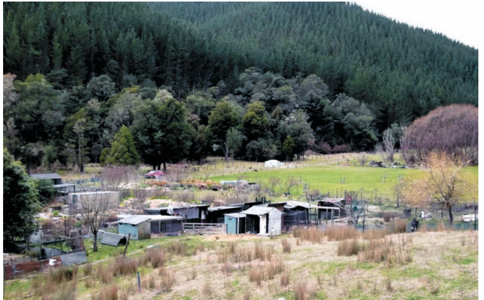
The solar pumping system provides water for the house, the veggie garden and chooks on this off-grid 20 ha property on the South Island of New Zealand.
