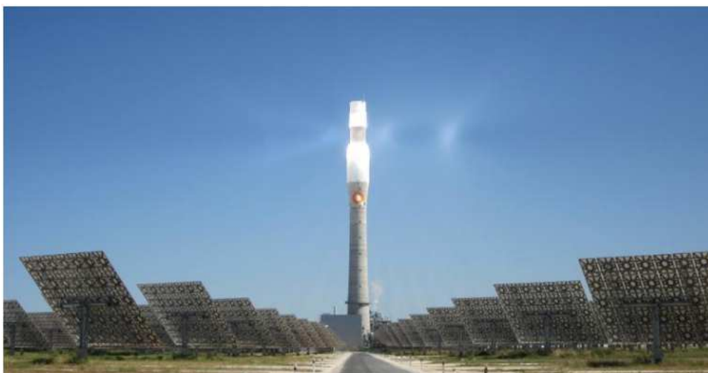
Figure 7: Concentrating solar thermal power station.
