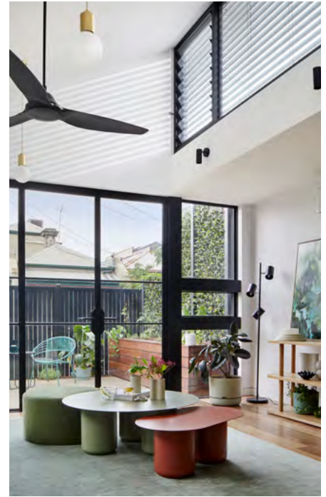
↑ High windows to the north bring in sunlight and warmth, and are equipped with mechanised external blinds for shading in summer.
