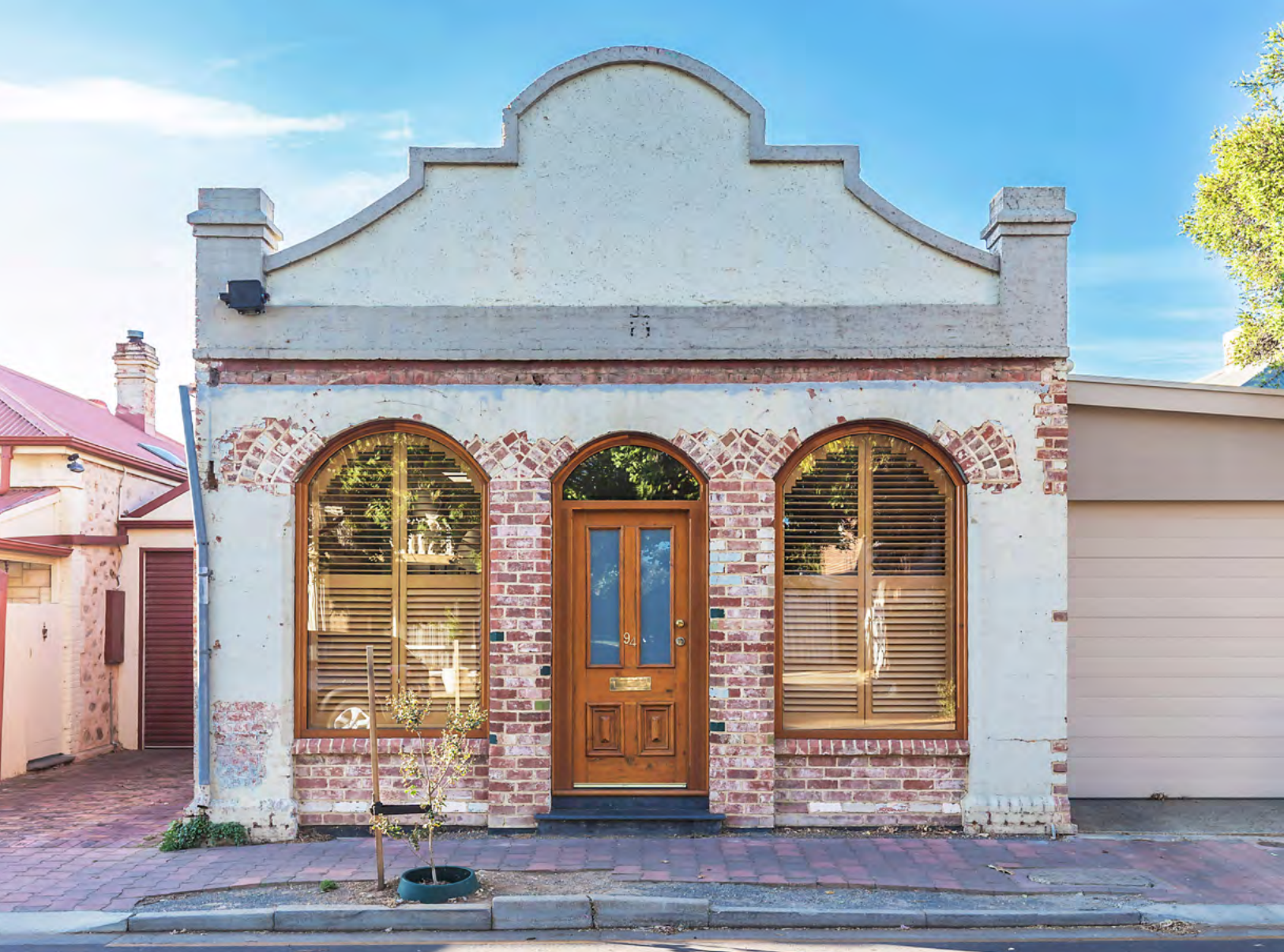
↑ The facade of the shop was restored to its original design, based on an old photo unearthed by the homeowners.
