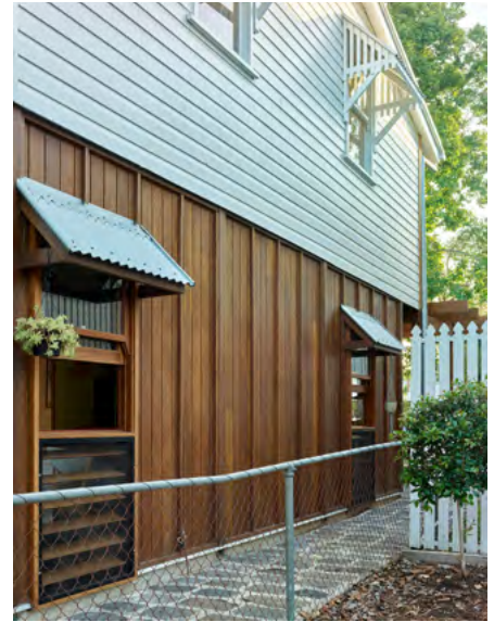
↑ The external walls downstairs have been designed to eliminate cavities within where water could accumulate, using hardwood framing and cladding with extruded polystyrene insulation.
