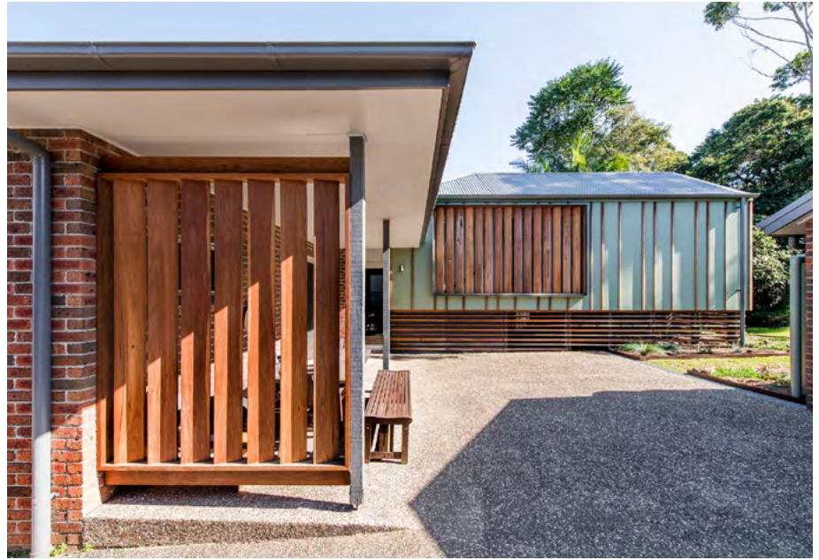
↑ Slatted timber screens provide shade and privacy to the patio and the east facade of the extension.
