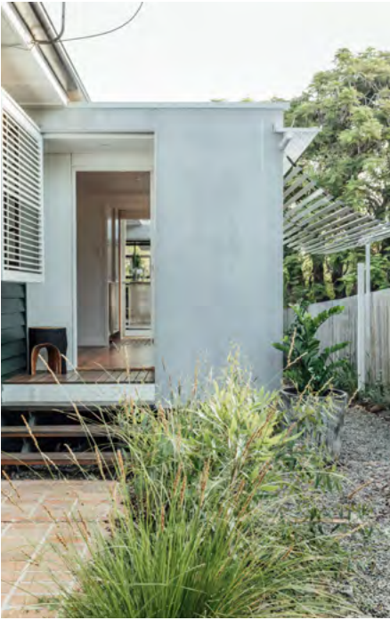
↑ A small addition to the western side of the house extends the living space and accommodates a laundry. Louvred 'vent boxes' to existing windows and adjustable slatted awnings provide shade.
