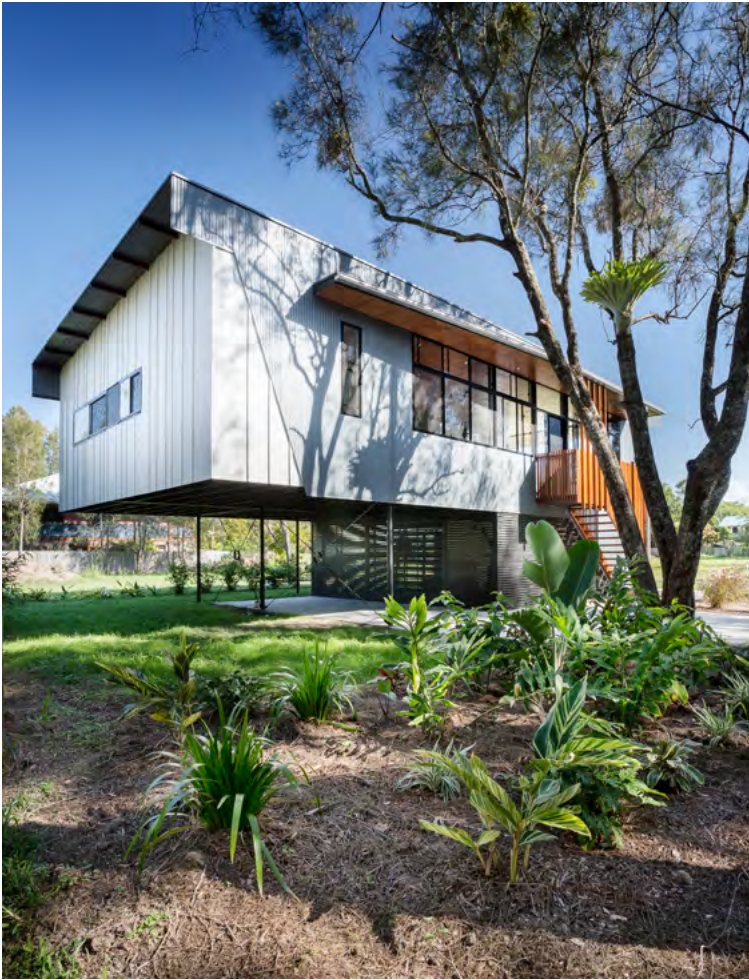
↑ A small undercroft houses garage, laundry and rainwater tank, and is built with one blockwork wall for bracing and other walls of hardwood timber slats to allow floodwater to flow through and air to circulate.
