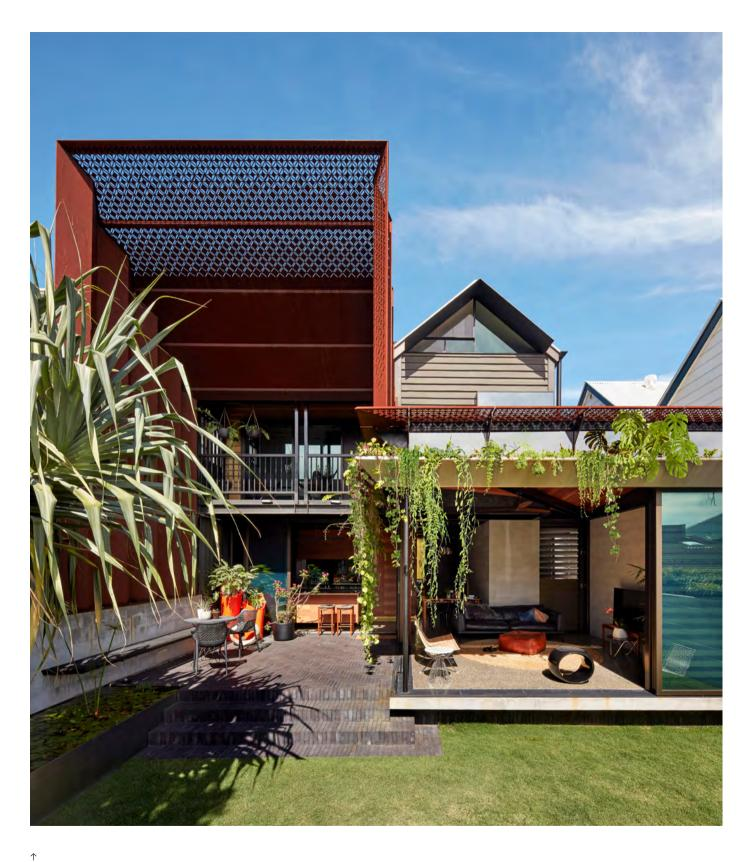
While the building now has a solidity to it with all the concrete and steel, "there are lots of delicate things happening", says architect Brian Steendyk of his renovated workers cottage. The soaring Corten steel awning is folded for stiffness, its edges perforated to create negative pressure in wind and to throw intricate shadows.
