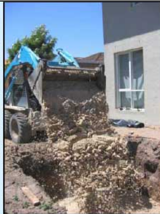
2. Filling sand filter – first layer.
