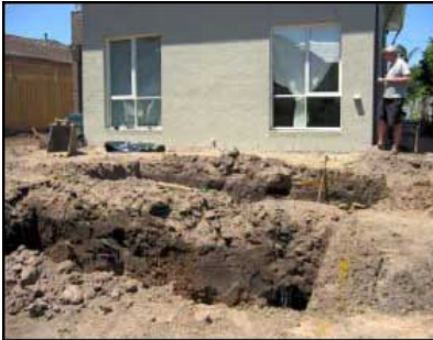
1. Pits are excavated for the sandfilter, pump wells and settling tank.
