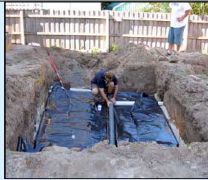
3. Paul Talbot lays the collection pipe to the base of the sand filter.
